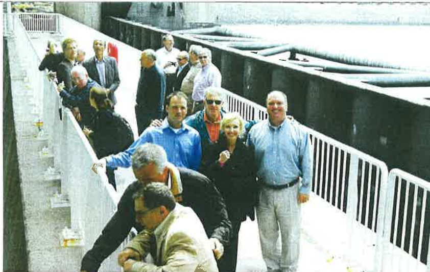
INSTITUTING A SOLUTION: As planning for a south Louisiana Water Institute continues, officials from the Baton Rouge Area Foundation and the Coastal Protection and Restoration Authority took a study trip to the Netherlands in June. Shown are CPRA deputy director Kyle Graham, BRAF CEO John Davies, BRAF consultant Christel Slaughter and BRAF legal counsel Edmund Giering visiting the Eastern Scheldt storm surge barrier.
